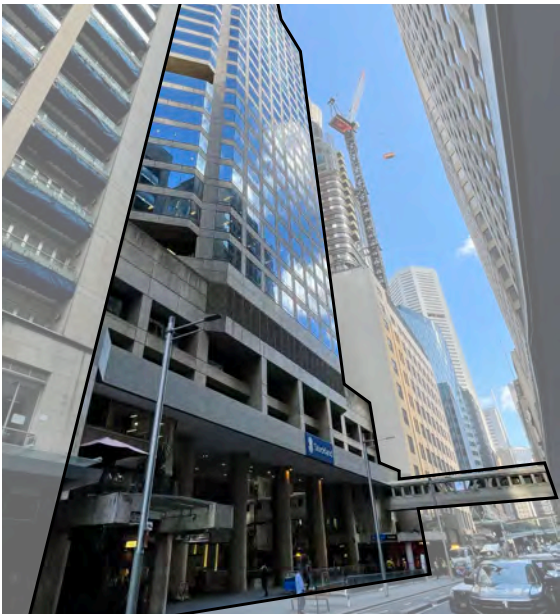
Existing view 1 - Site entrance from Castlereagh St.
